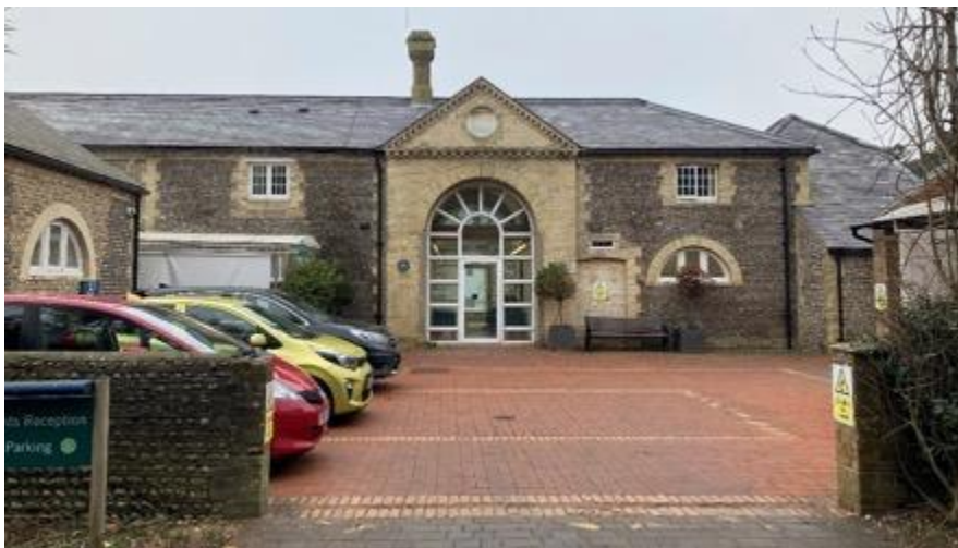
Figure 21: Former stable building at Goring Hall
