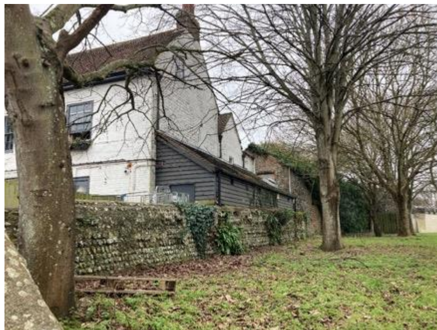
Figure 23: Examples of brick, flint and weatherboarding on and next to The Bull's Head.
